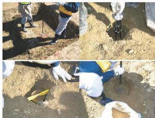
Fig.6 ワイヤレス間隙水圧計の設置状況 Views of setting up the wireless transducer
